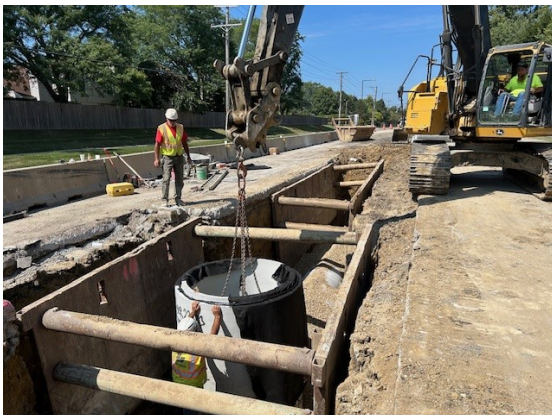
Manhole installation
