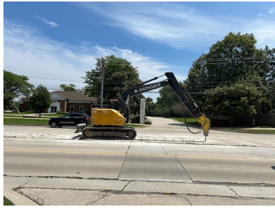
Median pavement removal on Arlington Heights Road
