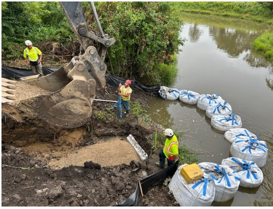
Storm sewer installation along Buffalo Creek
