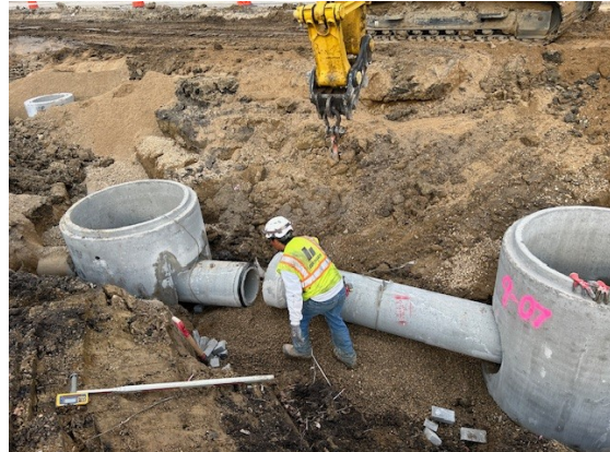
Storm sewer installation
