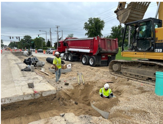
Storm sewer installation
