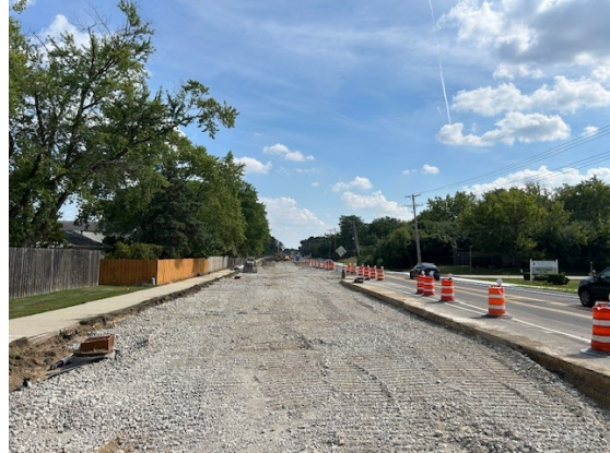
The first layer of the new roadway is being laid
