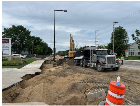
Pavement removal on the east side of Arlington Heights Road
