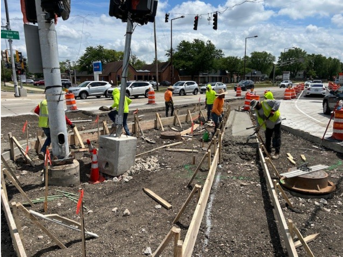
Pavement removal on the south side of Checker Drive
