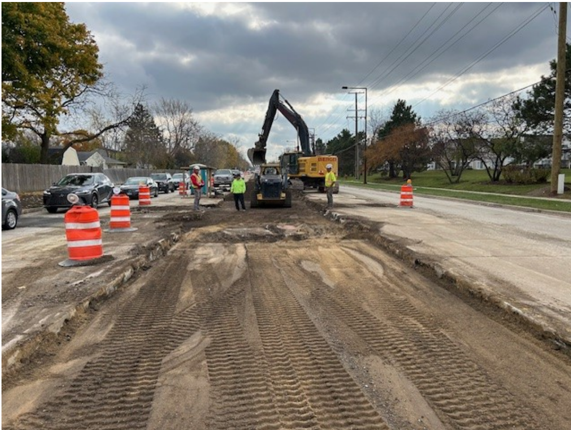
Median preparation for temporary pavement
