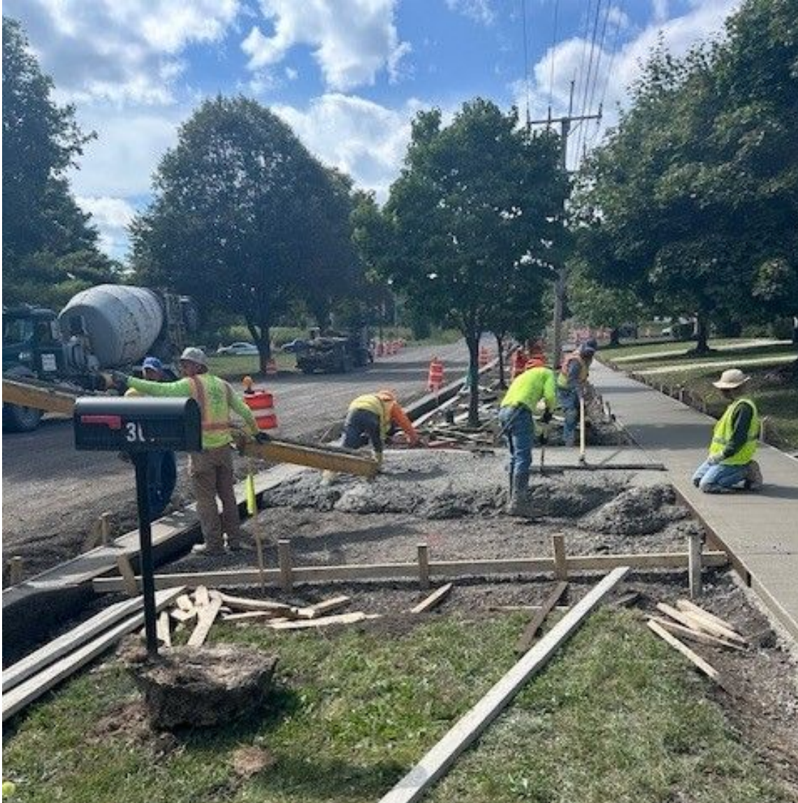
New sidewalk and driveway installation along Checker Drive
