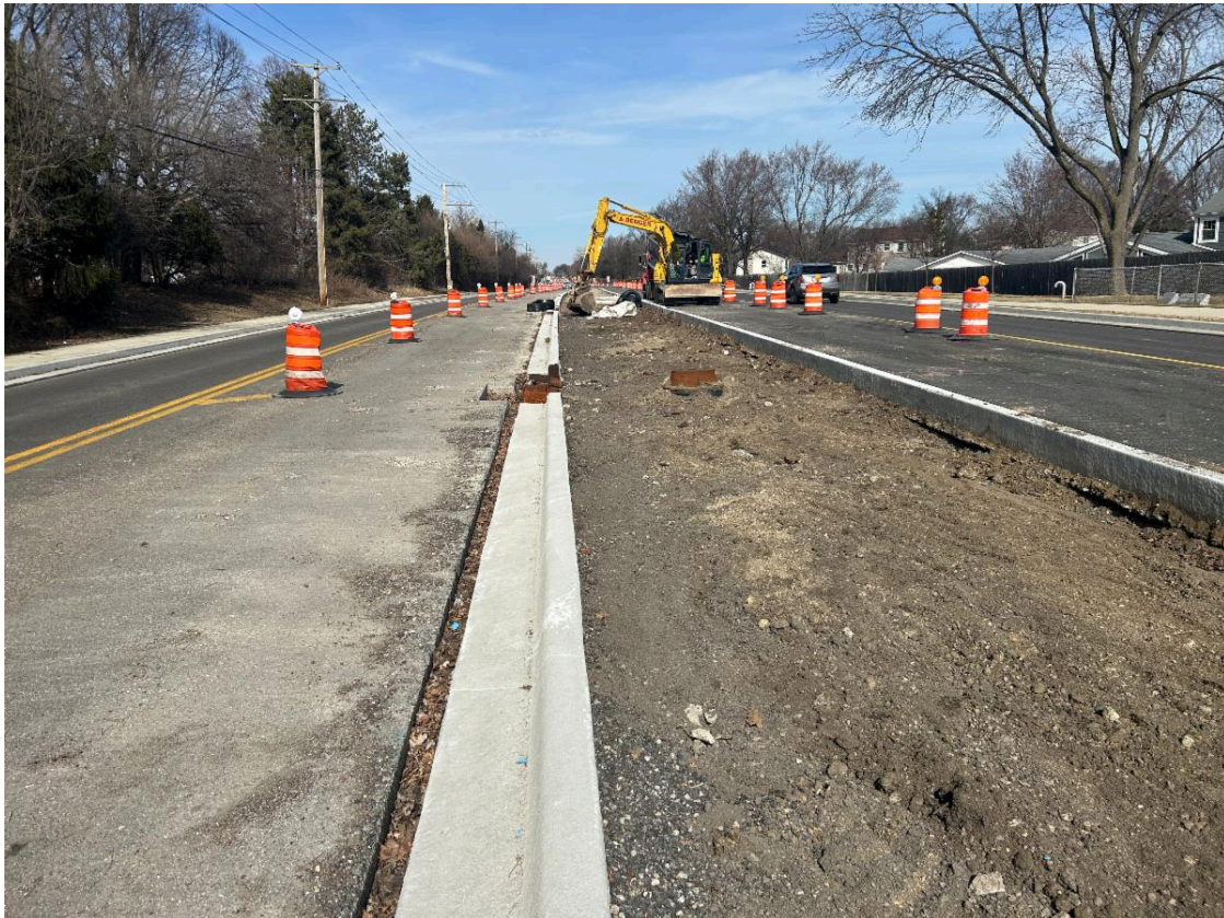
Prepping medians for topsoil along Arlington Heights Road!
